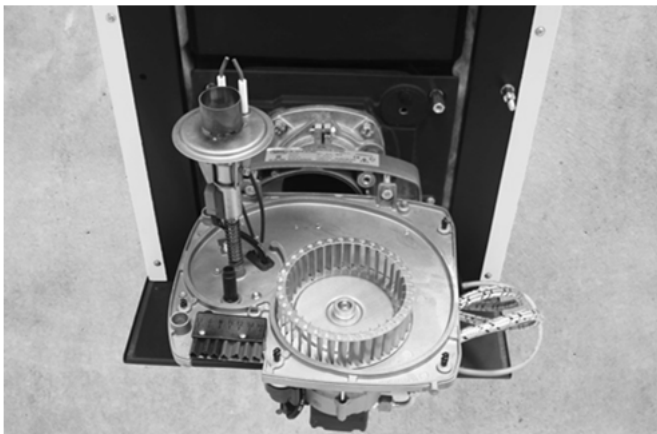
Abb. 32: Brenner in Serviceposition
